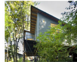
YELSER COMMUNITY CENTER View Project
